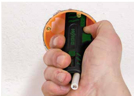
Stripping a cable sheath.
