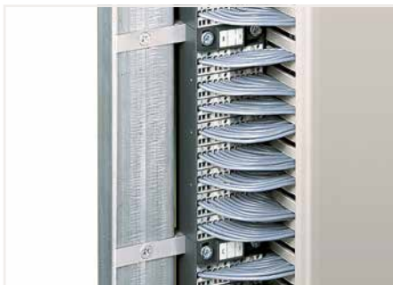
Installation example: Matrix patchboards in a frame
