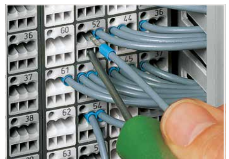
Terminating ferruled conductors via operating tool.
