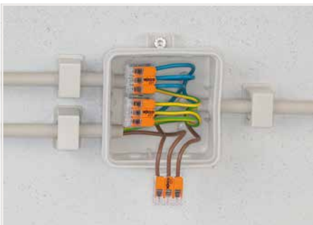
Wiring fine-stranded conductors in a junction box.
