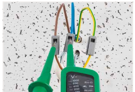
Testing via separate test ports.
