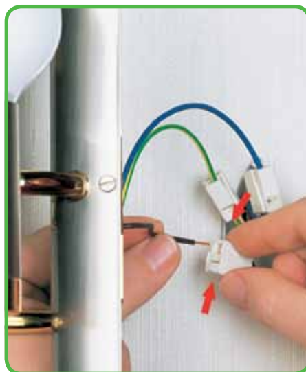
Testing through separate test slot
