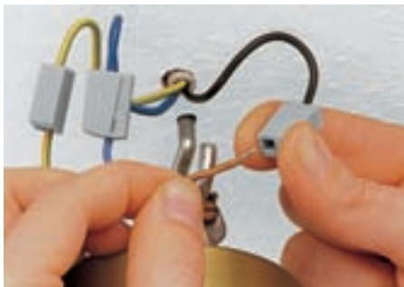
Connection of conductors (lighting side): Press button fully and insert stripped conductor into square entry and release.
