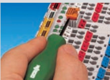
Function at locked position 1: Power output to I/O group is off
