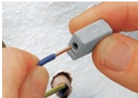
Connection of conductors (installation side): Introduce stripped solid conductor into circular entry and push to stop.
