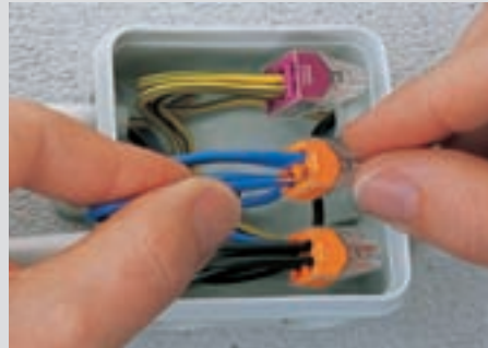
Connection: Insert stripped solid conductor FULLY
