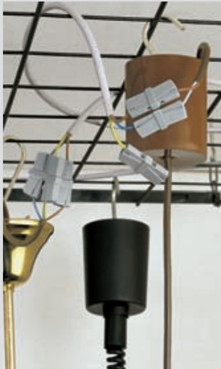
Wire connection: open clamping point using the lever and insert wire . . .
