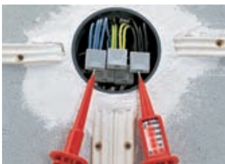
Voltage testing at push-wire connectors
