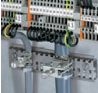
Mounting on a special slotted carrier rail
