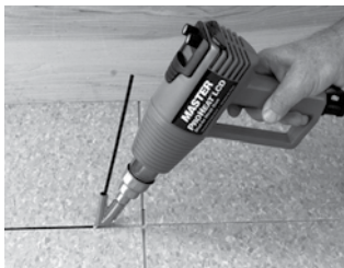
Welding Flooring Material
