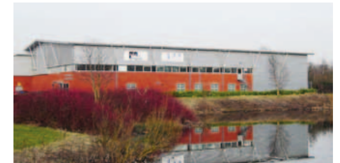
UK Distribution Centre, Warrington
