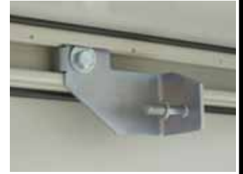
Secure bottom panel supports and upper panel mounting brackets into place. Upper panel mounting brackets feature a heavy duty collar stud. Notches in strut provide locating guidance.
