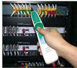
Copper cabling detecting
