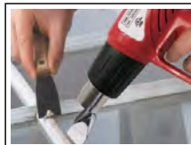
Removal of window glazing
