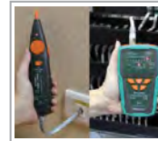
Verify LAN/ telephone cable condition
