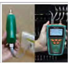
Verify LAN/ Telephone/ Coaxial cable condition
