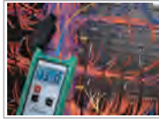
Fiber optic power test
