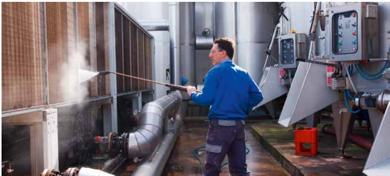
High-pressure wash down
